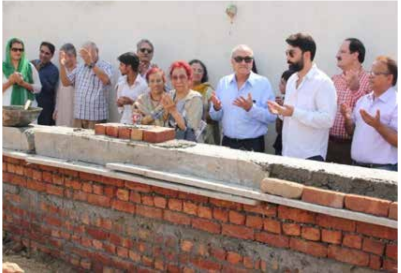
Mr. Zafar Bhatti in the centre, along with his son Mr. Babar Bhatti, with the Roshni Team at the foundation stone-laying of the new GERS building
